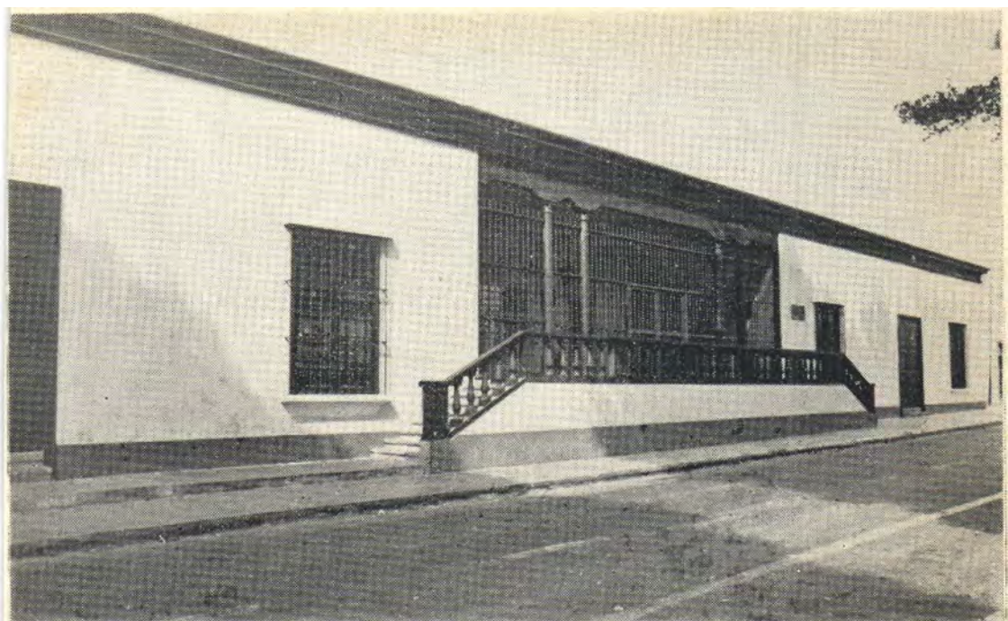
Fachada principal restaurada
